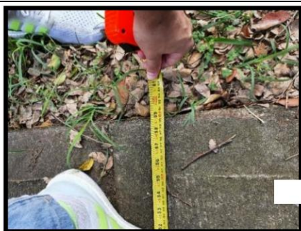
Figure 1 sidewalks of 150 cm in the area.
