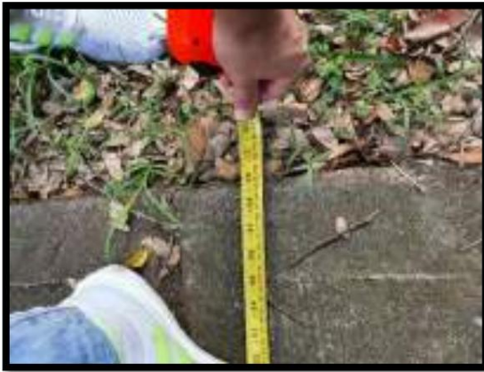
Figure 68 sidewalks of 150 cm in the area.
